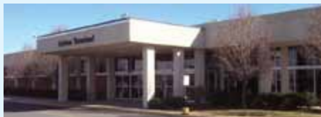
Shenandoah Valley Regional Airport
